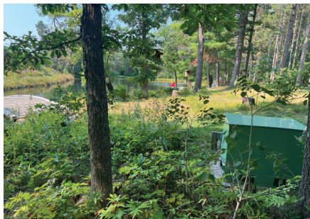
Figure 2: The Clear 50 nanobubble generator is shore-mounted and quiet.
