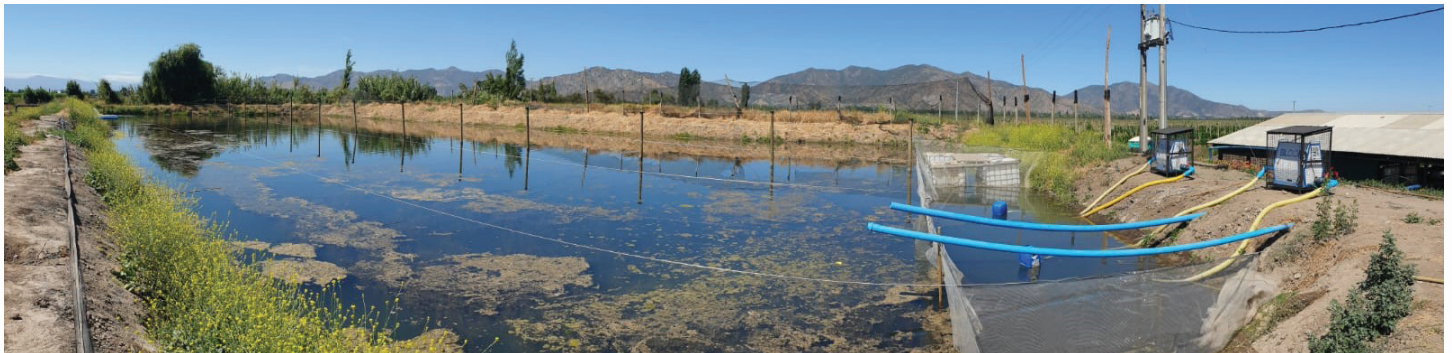
October 2020, at the installation of the nanobubble generator
