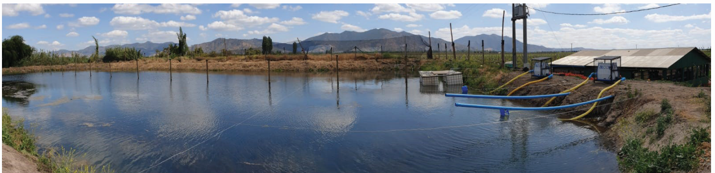
February 2021, 4 months after the installation
