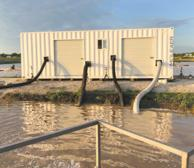
A food processing facility with a roughly 3-million-gallon wastewater lagoon was overloaded with solids, resulting in high effluent chemical oxygen demand (COD) and biochemical oxygen demand (BOD) concentrations. Using nanobubble technology, they were able to reduce effluent COD concentrations and degrade excess sludge that had accumulated in the lagoon..
