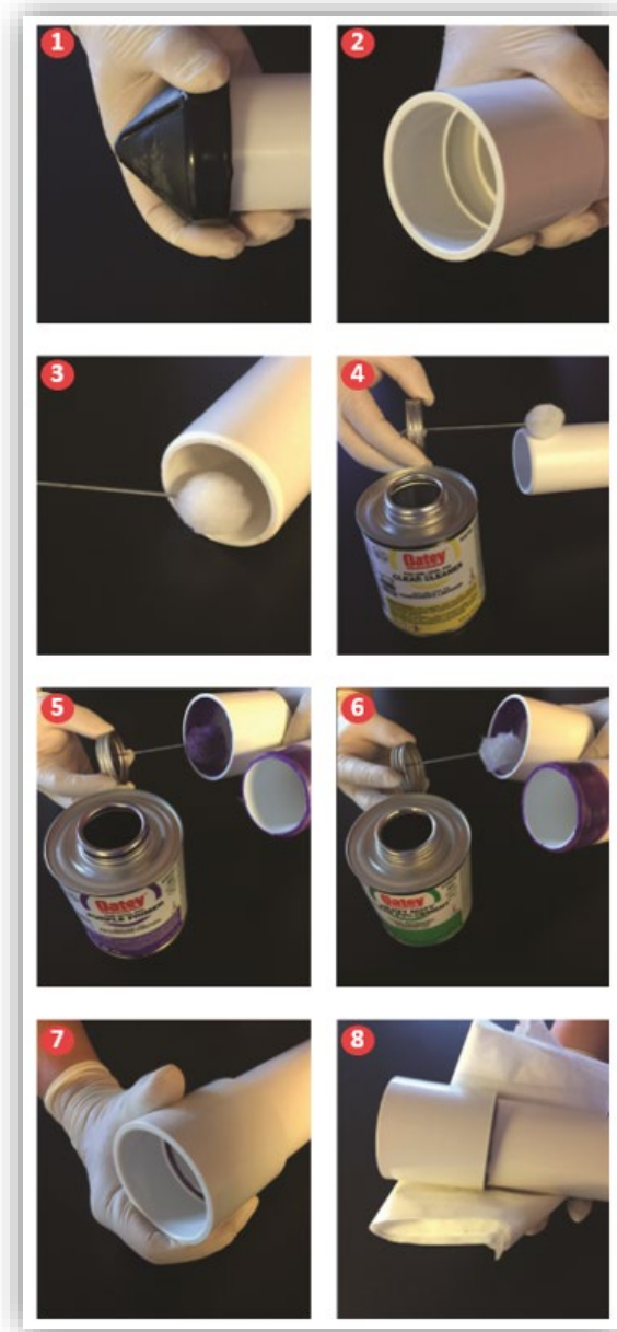
Figure 14. How to Glue Piping
